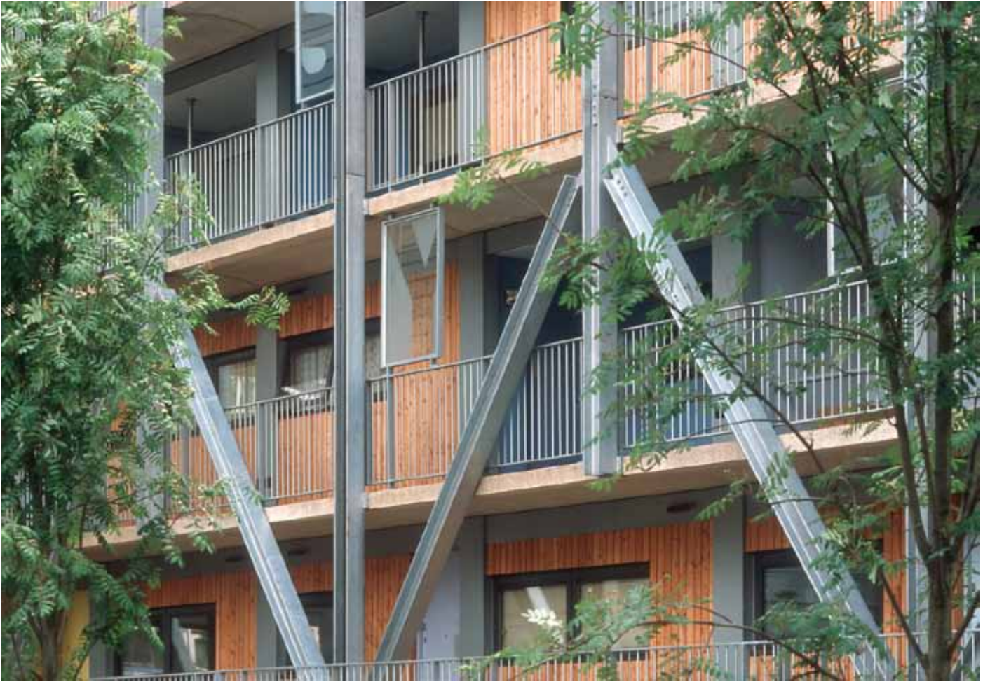
Access walkways to north elevation.
