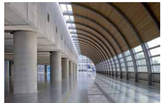
Tooley Street: Barnham Street barrel vault
