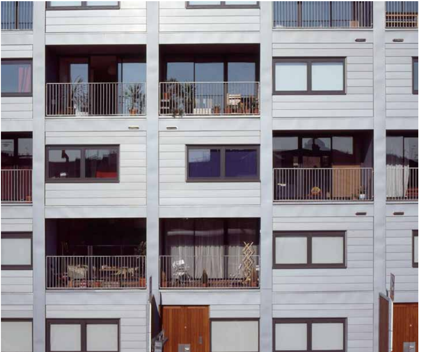
Zinc cladding and recessed balconies
