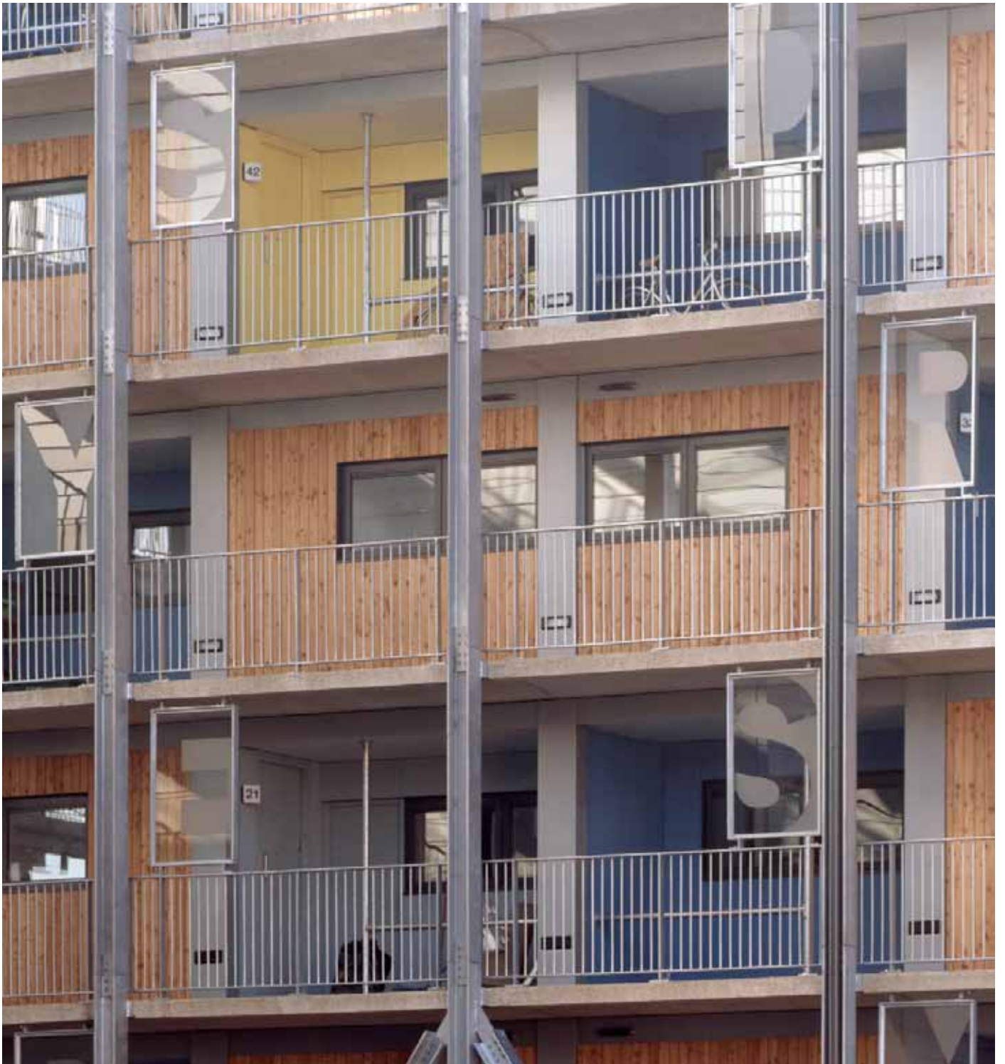
Access walkways to rear of site.
