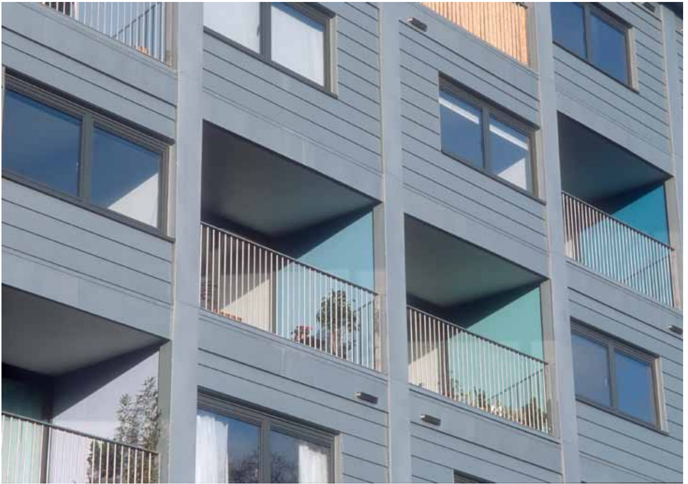
Zinc cladding and recessed balconies
